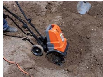
Figure 14. Digging the hole with a small tiller or "garden weeder"
